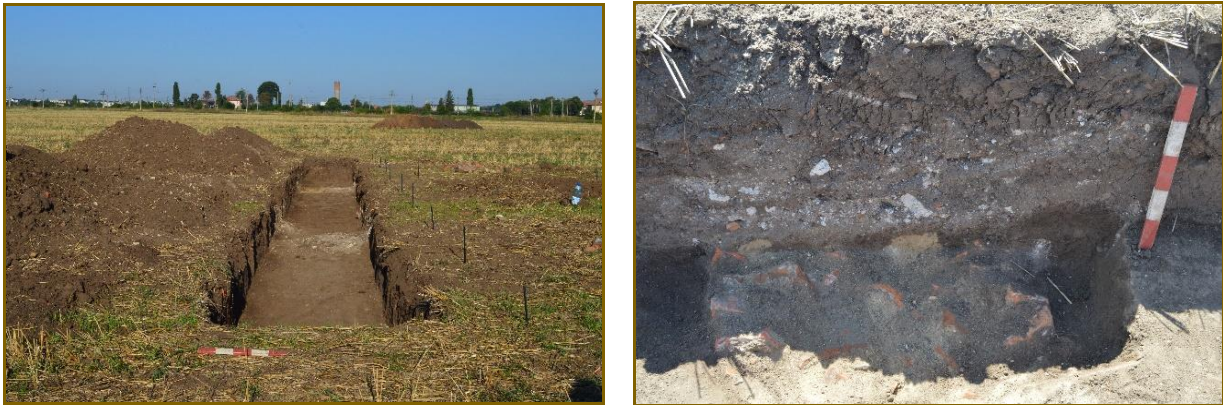
Figure 2. Caracal-Ring Road. Roman edifice No 1. General and detailed picture of the foundation
