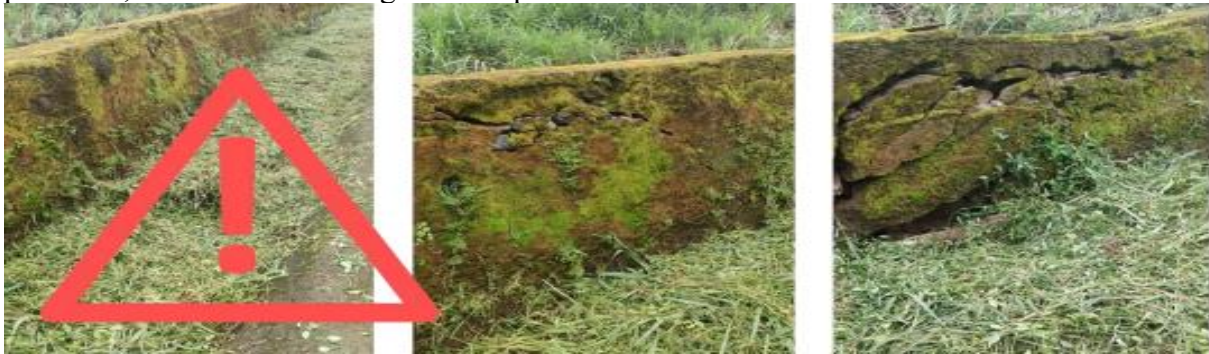
Plate 2: Evidence of protective wall collapse at the Zoological Center due to mismanagement
