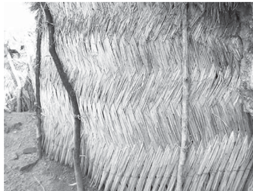
Figure D6: Gballi 'zana mat' used as a wall
